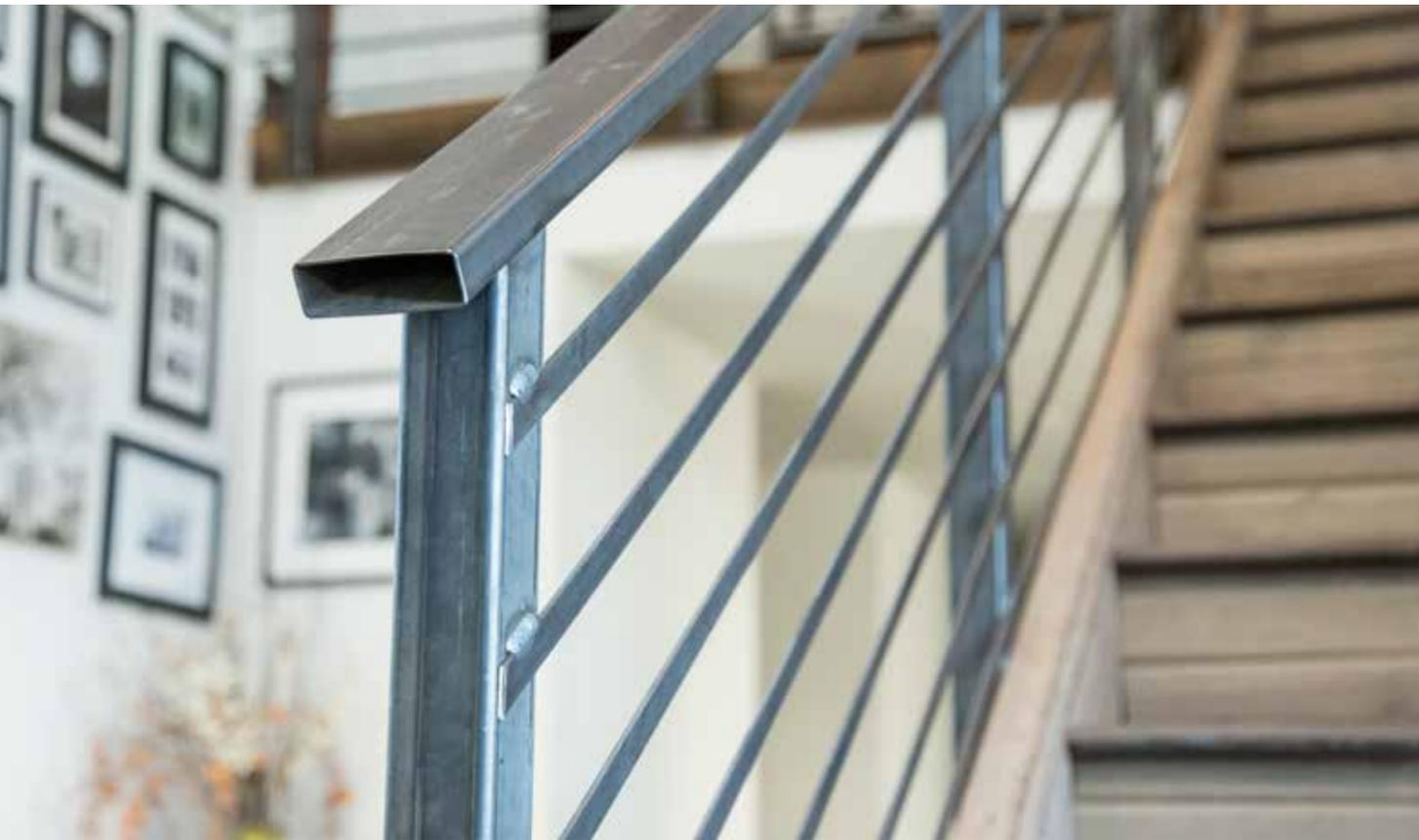
Steel stair rails were welded and built onsite.
